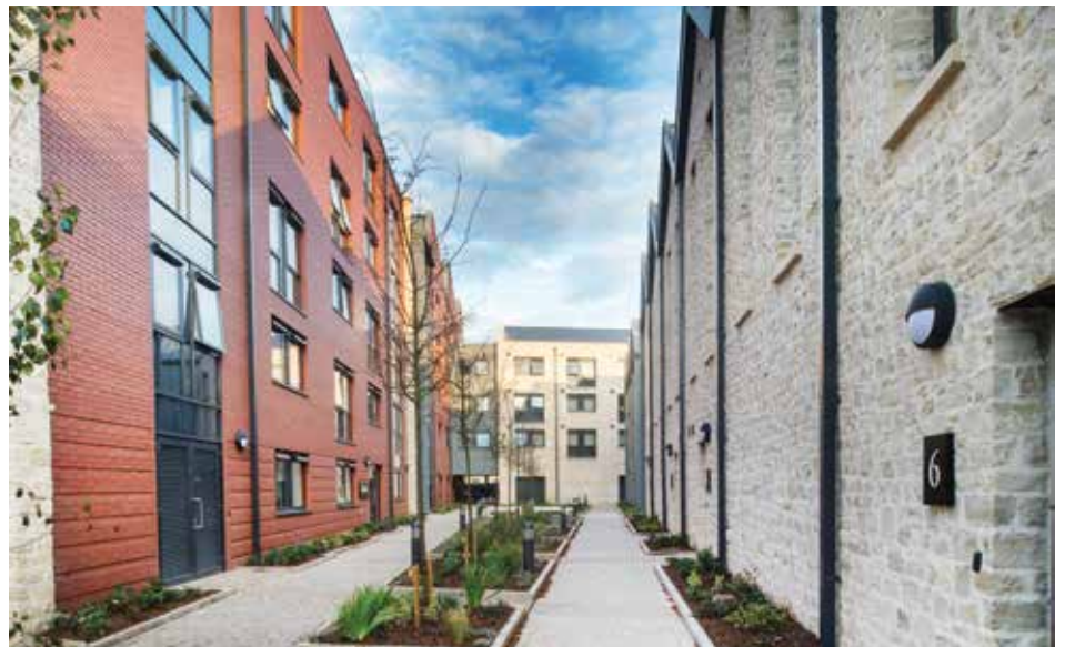
Twerton Mill – Internal courtyard demonstrating narrow site and linking buildings
